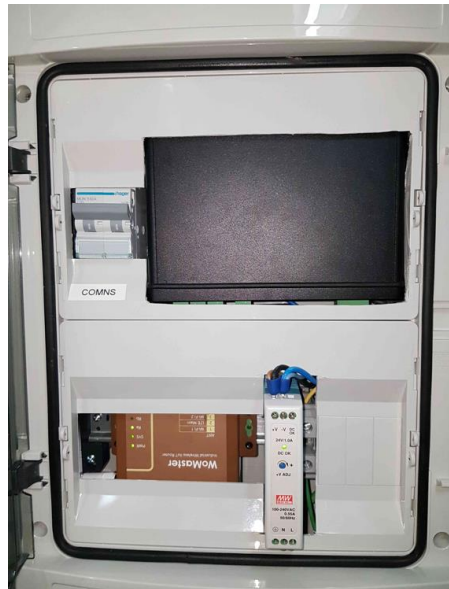
Figure 5 Energy Box installed at Málaga scenario
